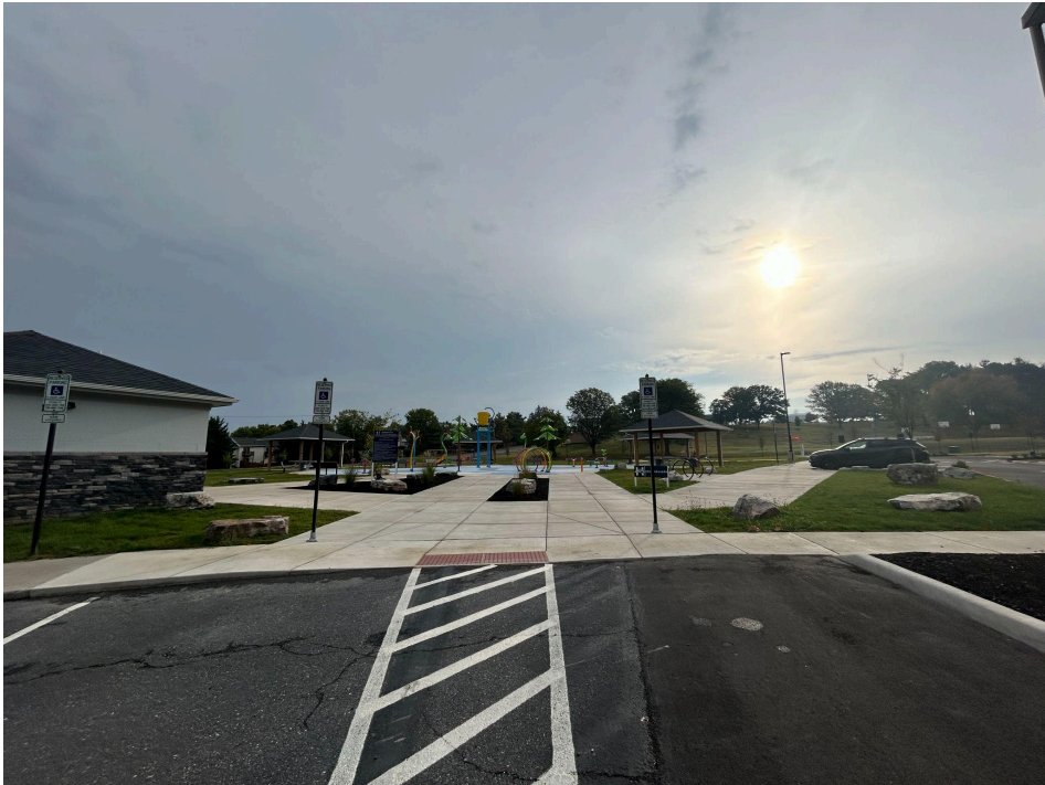
PHOTO OF SPRAYGROUNDS MAIN ENTRY, WHERE ARCHWAY IS TO BE LOCATED.
